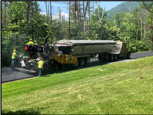
Paving work underway on Ways Lane, June 2025
